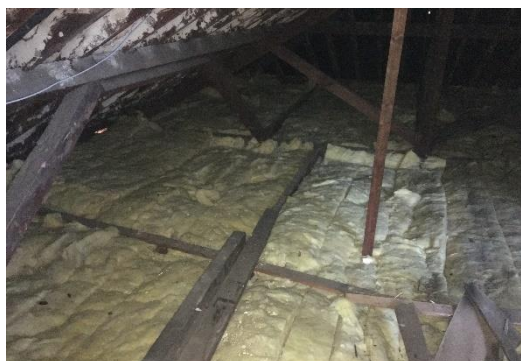
100mm insulation in the attic
