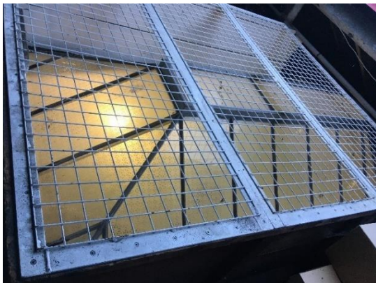
Decorative roof lantern to stairwell viewed from attic space
