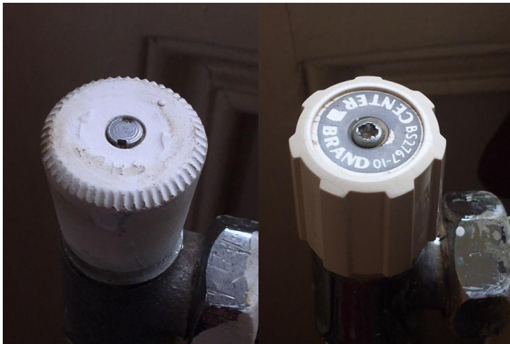
Examples of seized radiator flow and return valves
