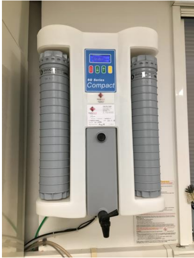
Upgrading point-of-use water treatment units at Geography
